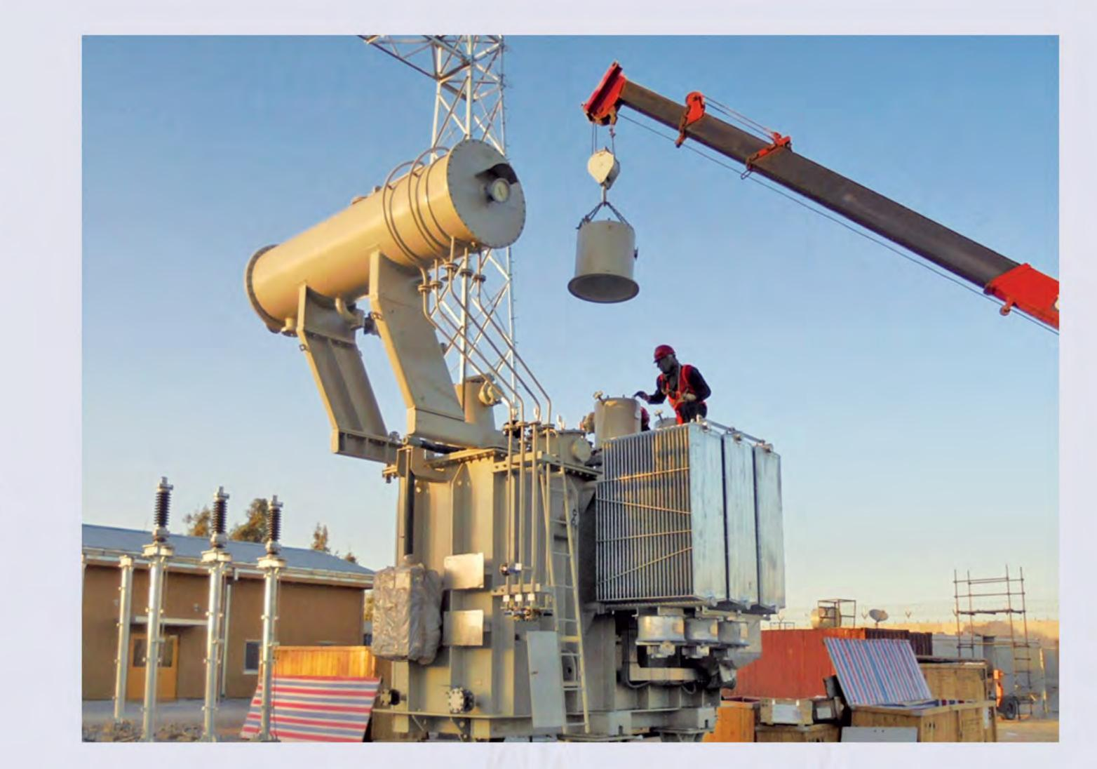
This is a project that will upgrade the high voltage power system in Kandahar, Afghanistan. Maiwand and Pushmol substations each shall have two 110 kV line bays, a 110/20 kV transformer rated no less than 20 MVA, a 20 kV yard with indoor switchgear. The objective of this project is to provide a cost effective, reliable power system for the distribution of electric power in Kandahar Province. Each substation shall be designed to support a 20 MVA transformer.
